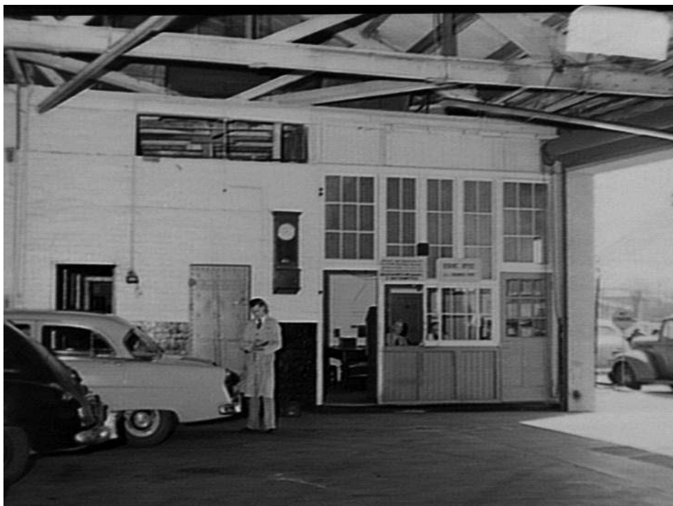
Figure 2.20 The administrative offices of 1913 building, which were located to the east of the two-storey section. Photograph is dated October 1953
