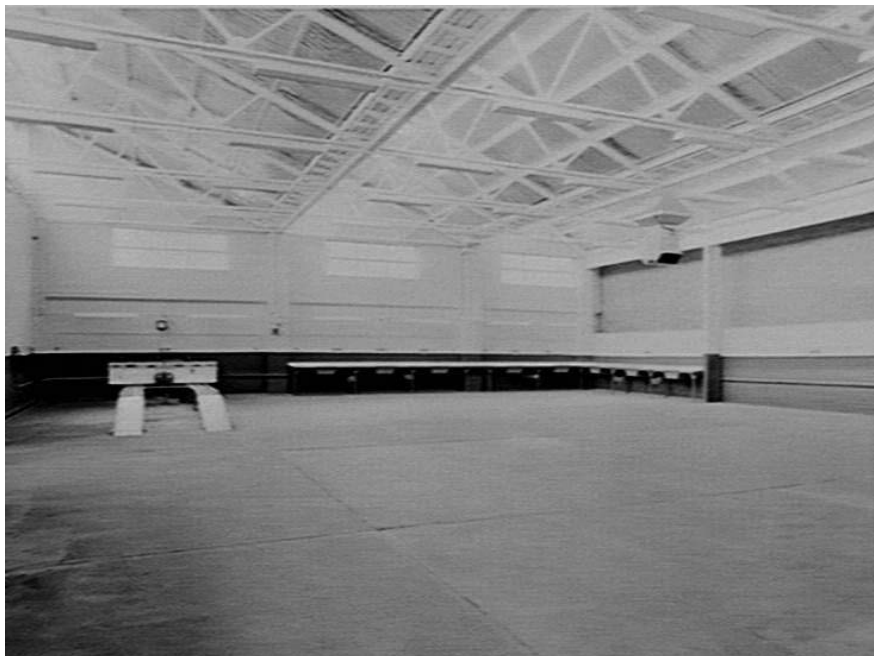
Figure 2.32 The interior of the 1947 extension refurbished in 1979. Photograph is dated February 1980
