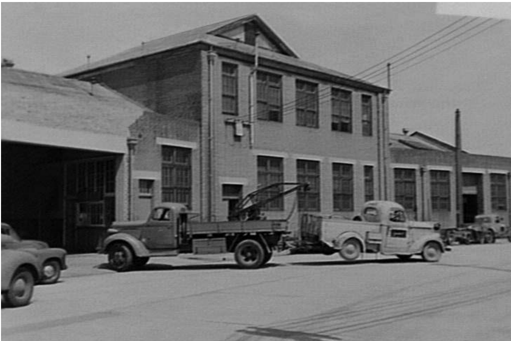
Figure 2.26 A detailed view of the crude door insertion, undertaken around 1947. Photograph is dated October 1953
